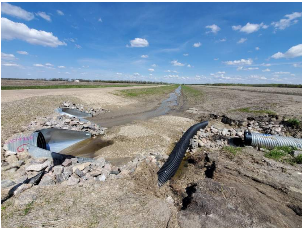
Site #23 – Erosion damage, culvert washed out, exposed subsurface drain tile line.
