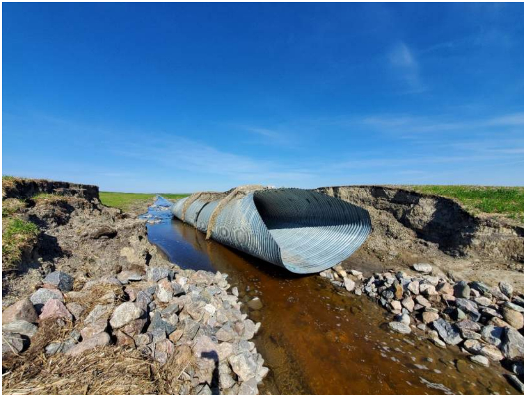
Site # 8 – Mainline pipe washed out.
