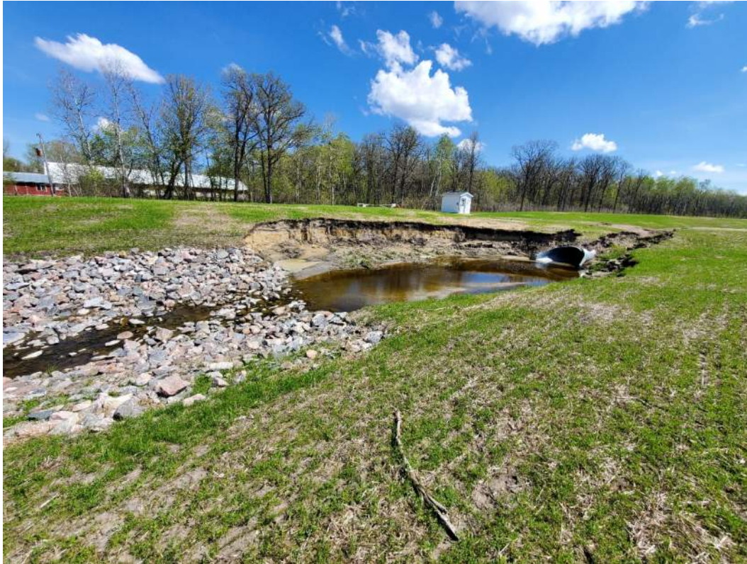
Site #17 – Mainline pipe and channel erosion.
