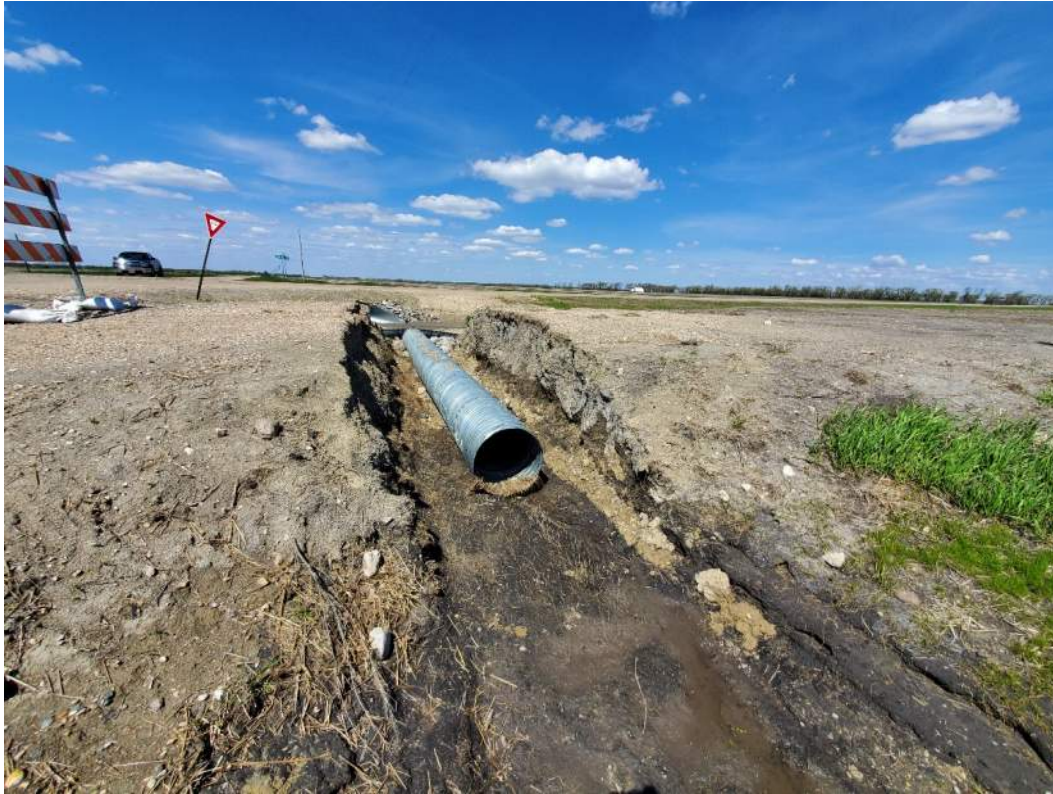
Site #23 – Culvert washed out.
