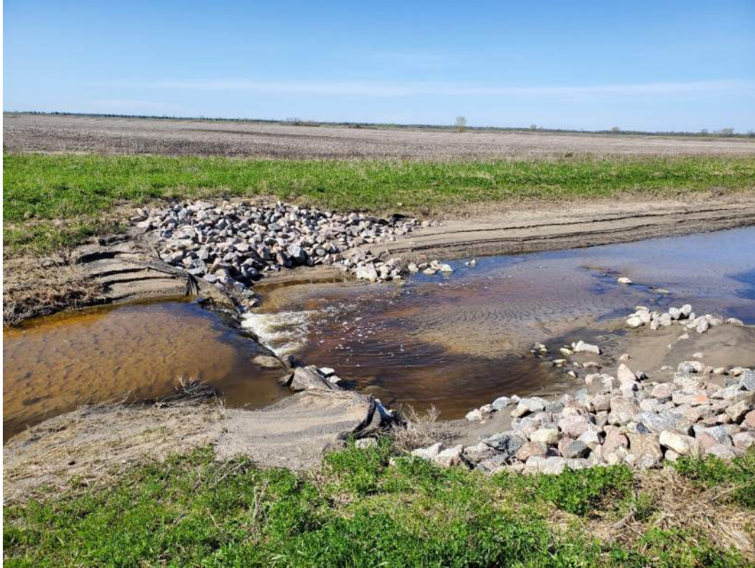
Site #6,#7,#9 – Rip rap displaced/eroded.
