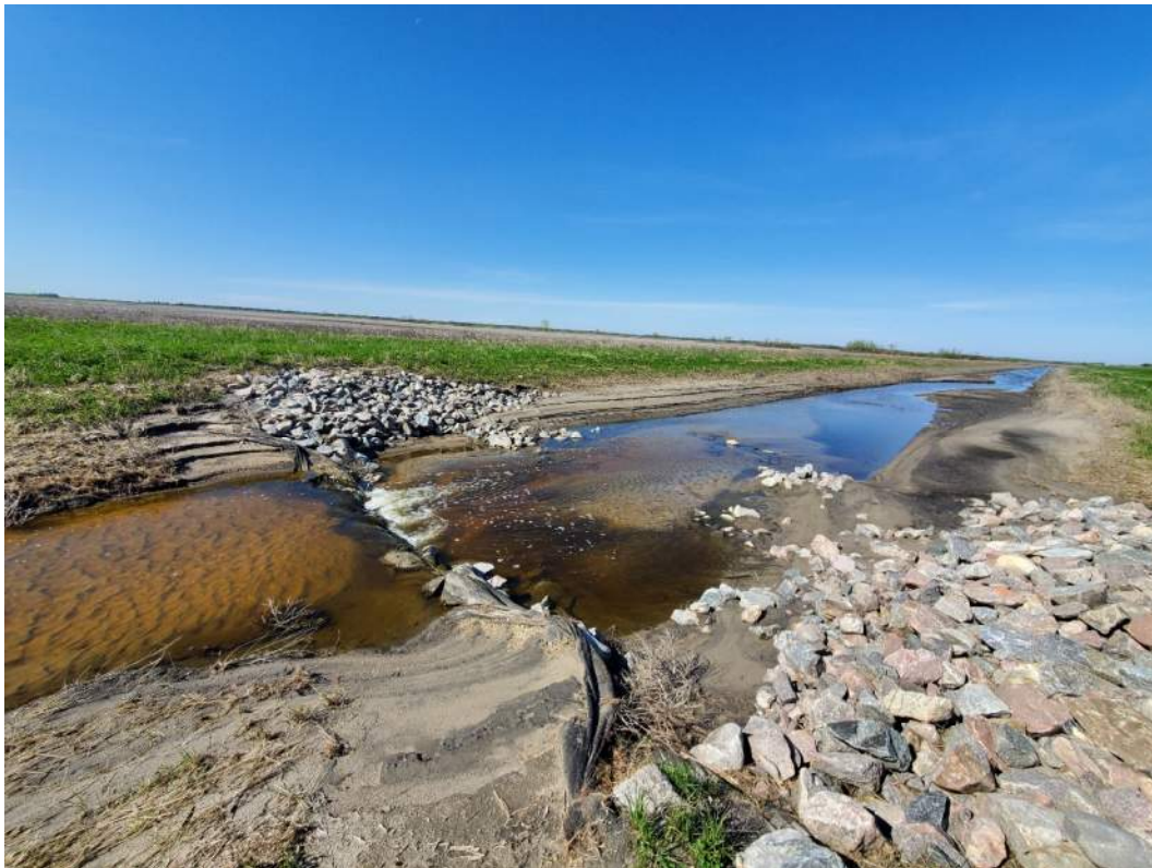
Site #11 – Riprap displaced eroded.
