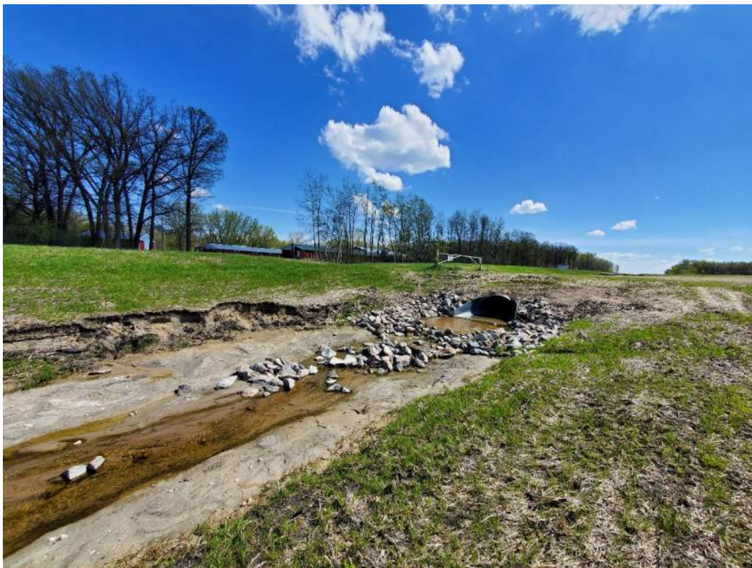
Site #16 – Mainline pipe and channel erosion.
