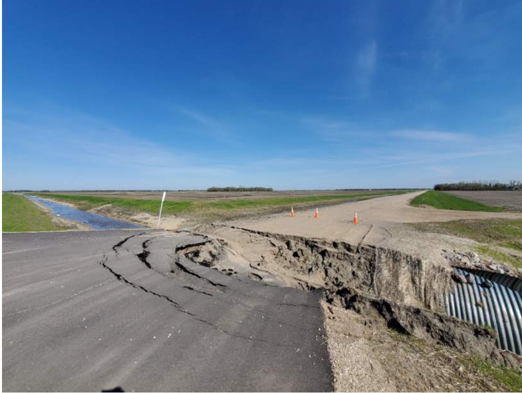
Site #10 – Mainline pipe washed out.
