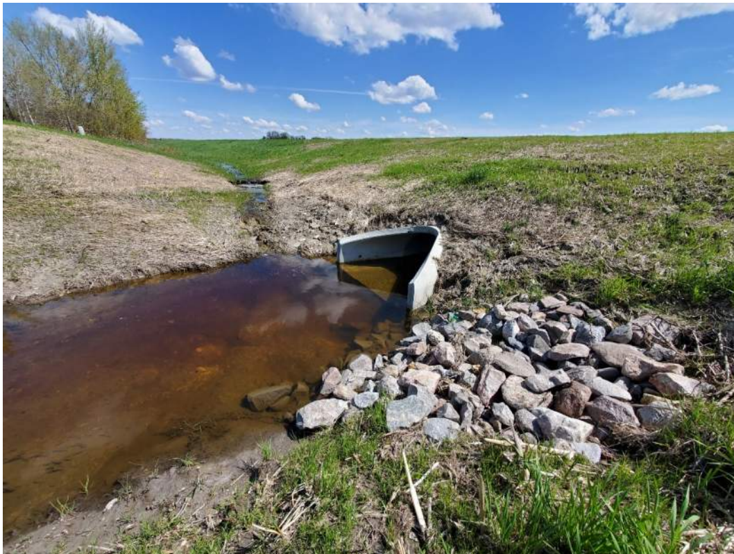
Site #20 – Erosion scour damage at outlet end of pipe.
