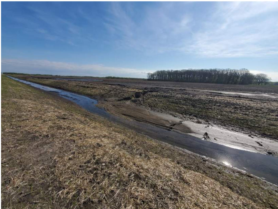
Site #2,3,4,5 – Erosion scour off field. Rock chute needed.
