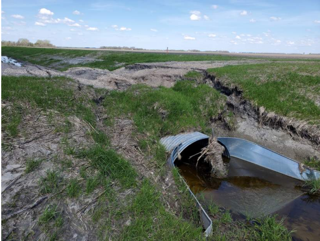
Site #14, 15 – Mainline pipe eroded.
