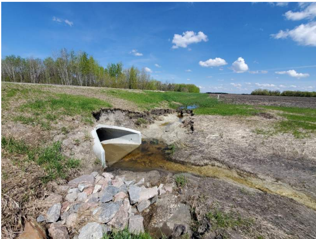
Site #18 – Erosion damage from highway ditch.
